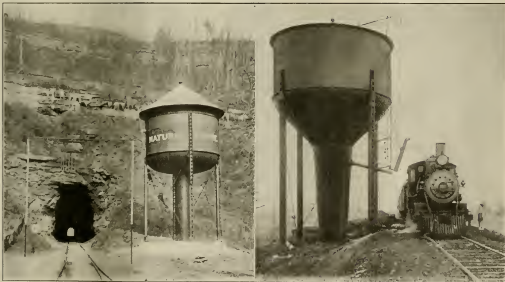
CONICAL TANK BOTTOM, L. & E. RY.
